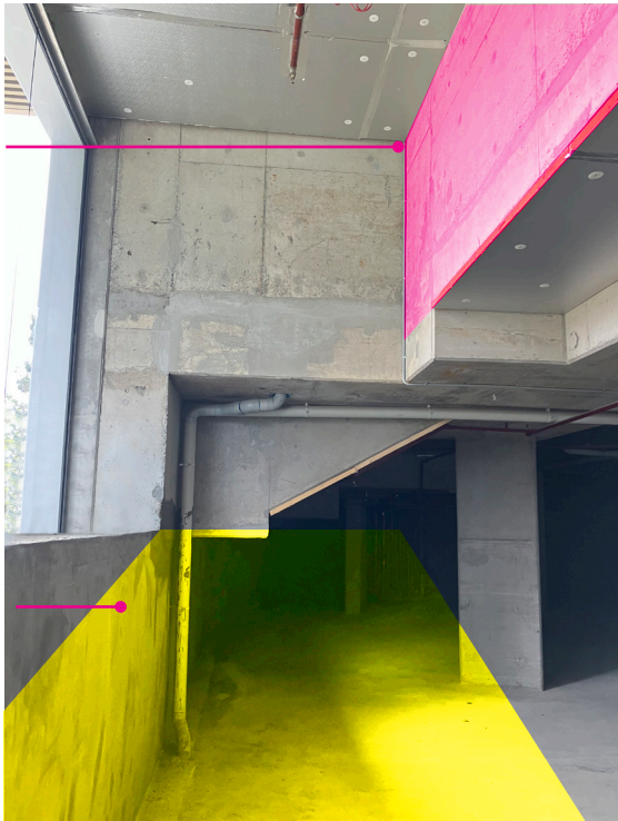
Bulkhead facing north west
