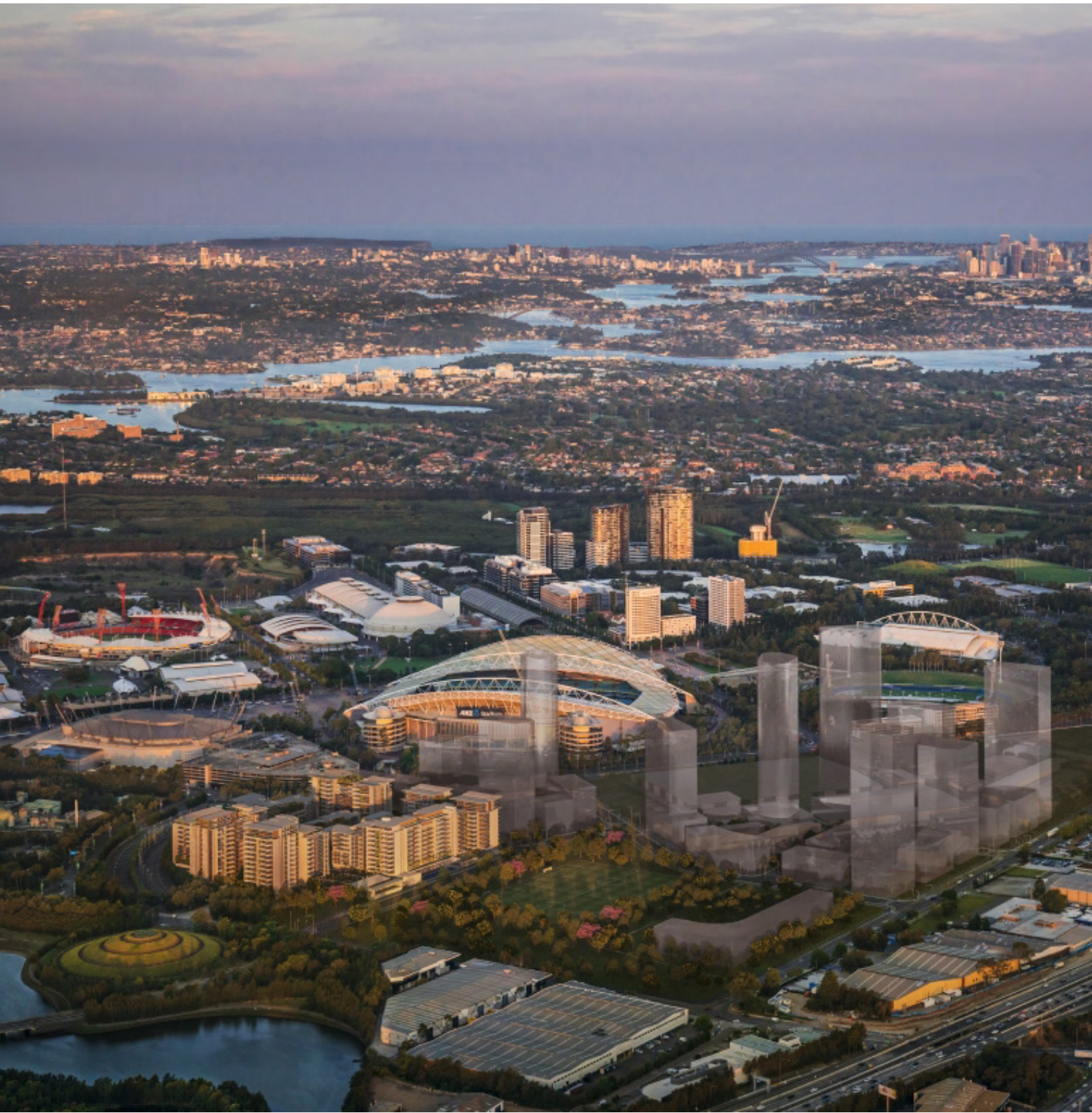
Revitalised Carter Street Precinct - NSW Department of Planning and Environment Masterplan for Carter Street Precinct, 2017. Article by The Urban Developer Fri 5 October 2018
