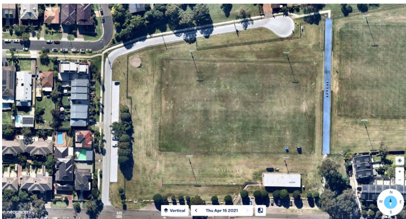
SUPPLEMENTARY IMAGE 4: Cool Roads Trial site at Corry Court, North Parramatta. The image shows both, the residential street and the carpark sites. Image was taken on 3 April 2021. © Nearmap.
