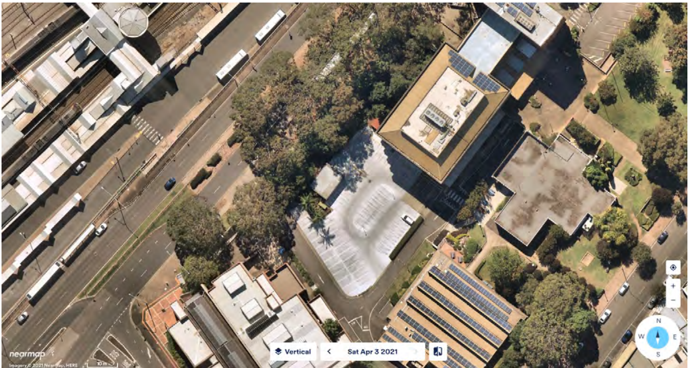
SUPPLEMENTARY IMAGE 5: Cool Roads Trial site at the Civic Centre, Hurley Street, Campbelltown. Image was taken on 3 April 2021. © Nearmap.
