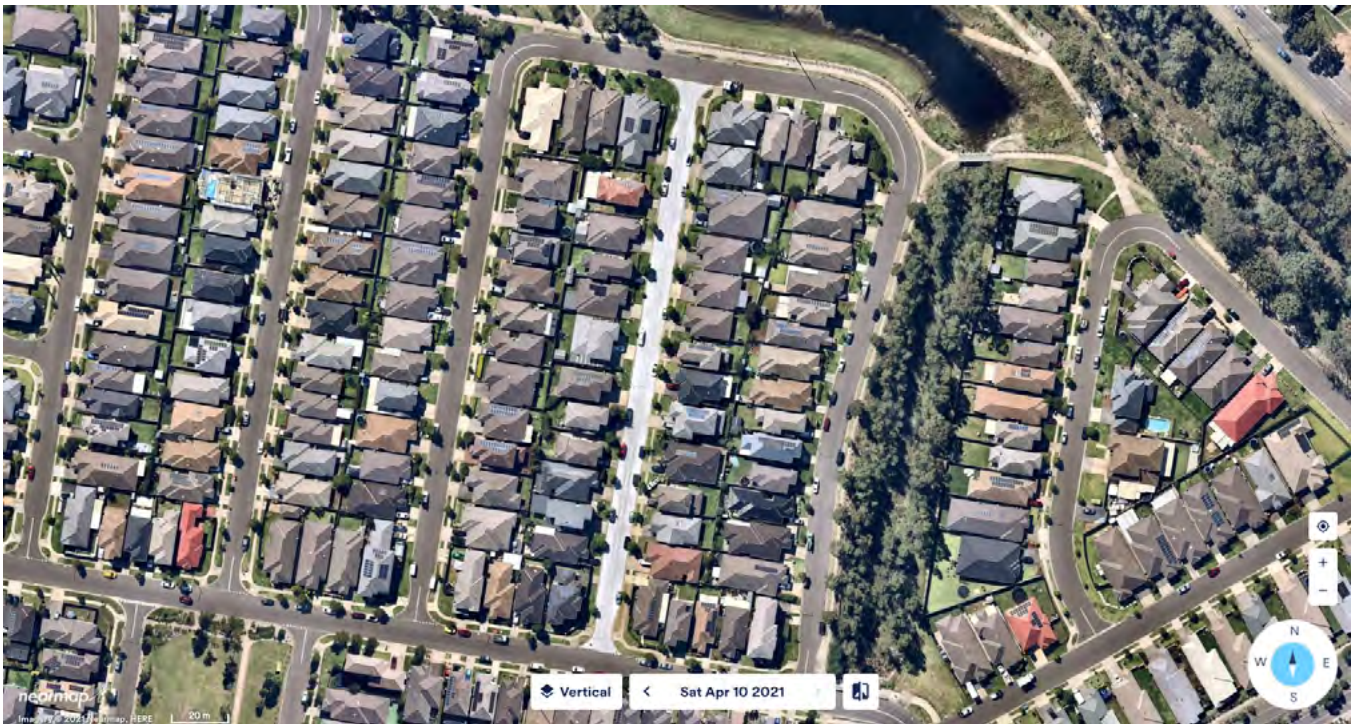
SUPPLEMENTARY IMAGE 8: Cool Roads Trial site at Kobe Street, Ropes Crossing. Image was taken on 3 April 2021. © Nearmap.
