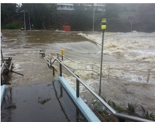
Charles Street Weir - April 2015
