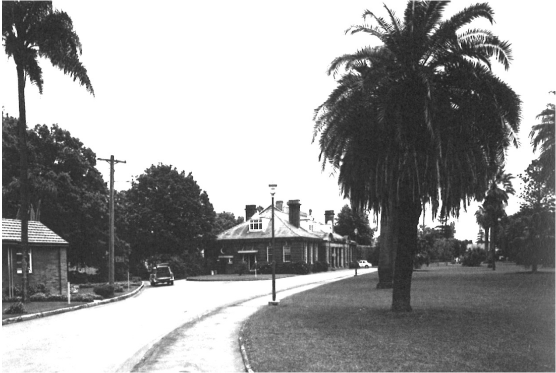
A-14 A January 1962 photograph of Greenup Drive leading towards the 'Administrative Offices'. This view is unlikely to have changed much since the building was first completed 50 years earlier, other than the maturation of the plantings. Source: Government Printer, Image 19027.
