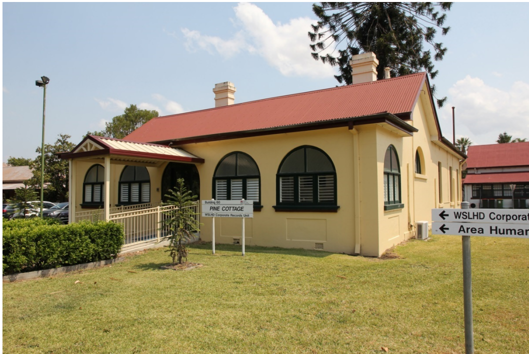
C-14 The east elevation/ entry of Pine Cottage showing the current signage, plantings and ramp. Source: TKD Architects, 2016.
