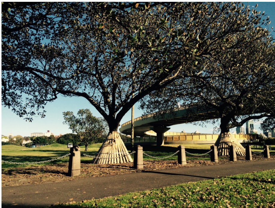
Figure 12 Trunks of mature figs protected by skirts of timber staves in Moore Park, beside the Albert (Tibby) Cotter Walkway pedestrian bridge. (Photo: Margaret Betteridge, 28 September 2015)
