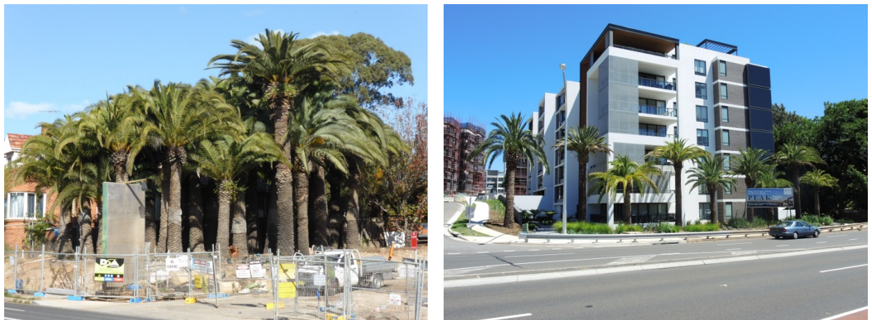
Figure 13 (Left): Specimens of Phoenix canariensis (Canary Island Date Palm) stored on site at Peak apartment development on Victoria Road, Ryde; (Right): Some of the specimens transplanted to landscape the new development. (Photos: Chris Betteridge, 21 July 2015 and 24 February 2016)
