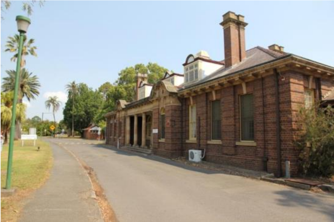
A-21 The east elevation of the Mental Health Sciences building. Source: TKD Architects, 2016.
