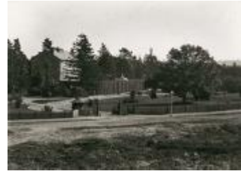
The c1904 entry facilitated by the resumption of the residential property along Fleet Street.
