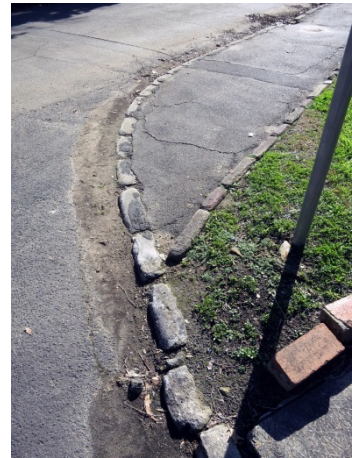
A remnant section of sandstone kerbs and path edging on Eastern Circuit that extend across the Public Domain
