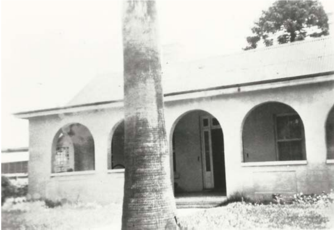
C-6 The 1943 image shows the infill of the verandah and maturation of one of the bunya pines planting in the eastern courtyard of Pine Cottage. Source: Cumberland Hospital Museum.
