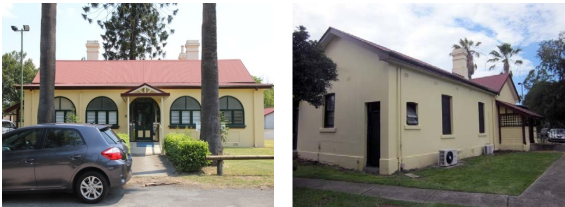
C-16 The main entrance to Pine Cottage showing porch addition and mature trees (left) and south elevation of Pine Cottage showing intrusive services, porch addition, circulation paths and mature trees (right). Source: TKD Architects, 2016.
