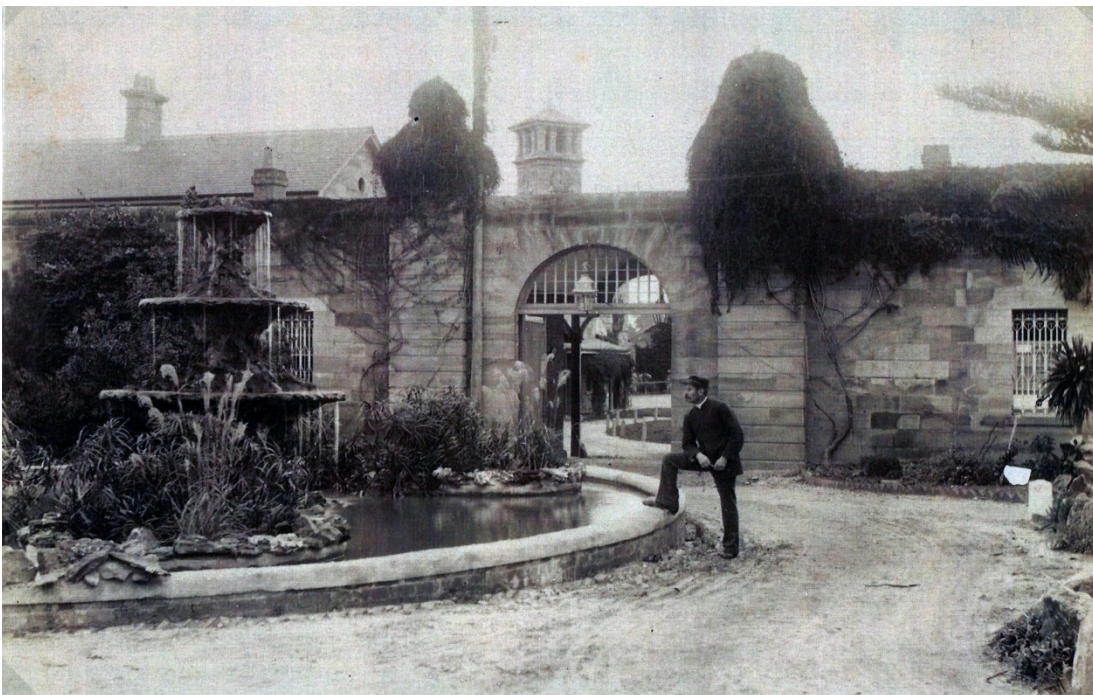
A-2 A c1888 photograph of the original entry to the Female Factory. The photograph was possibly taken to document the completion of the 'Fish Pond, Fountain & Rockery', which now dominates the entry to the complex. The clock tower of the c1884 dormitory building (Male Ward 1) is visible in the background. Source: tbc.
