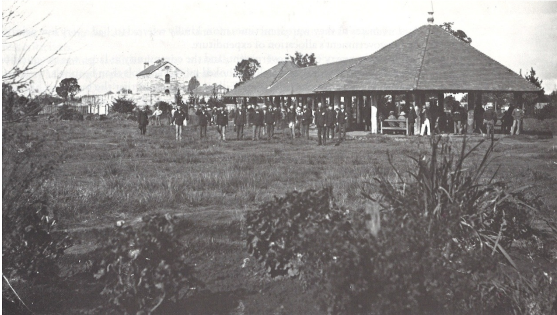
B-2 This 1880s image shows the Male Shelter Shed viewed from the north end of what became the Sports Oval. The structure's function as a social and recreational shelter is evident. Views of the wider setting can be seen, enabled by the structure's open character and form. Timber shingle roof cladding, pinnacles on both hexagonal wings and roughly-hewn timber posts are noted. Source: Parramatta Heritage Centre.
