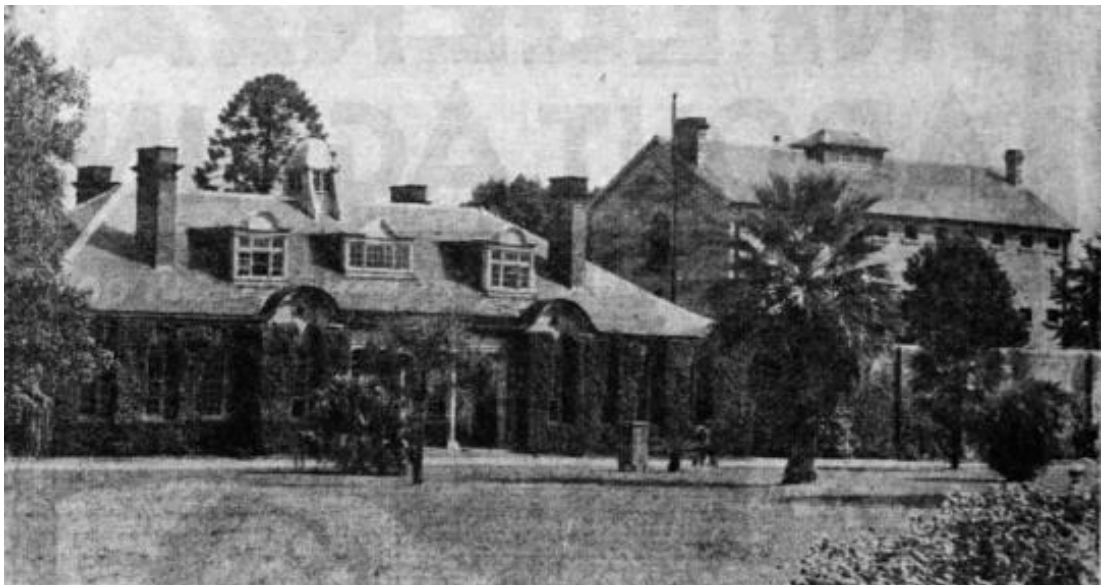
A-10 A 1936 photograph showing the east elevation of the 'Administrative Offices'. The stone wall and Criminal Lunatic Ward are to the right of the building. Source: Australian Women's Weekly, with TKD Architects overlay, 2016.
