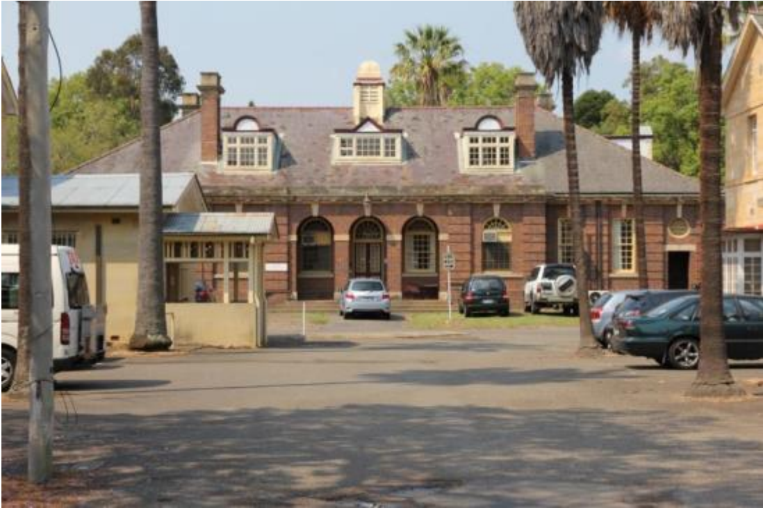
A-20 The west elevation of the Mental Health Sciences building and adjacent structures including the State Health Credit Union and the NSW Institute of Psychiatry buildings. Source: TKD Architects, 2016.
