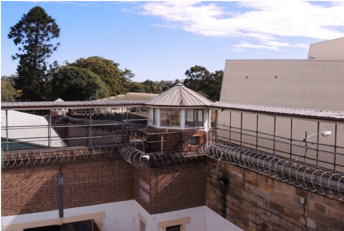
52 Guard Tower (Building P27) at centre with the view to the Guard Tower at the north-western boundary of the Gaol and the southern end of the Linen Service (Building L4) at right. Source: MUSEcape, October 2015.
