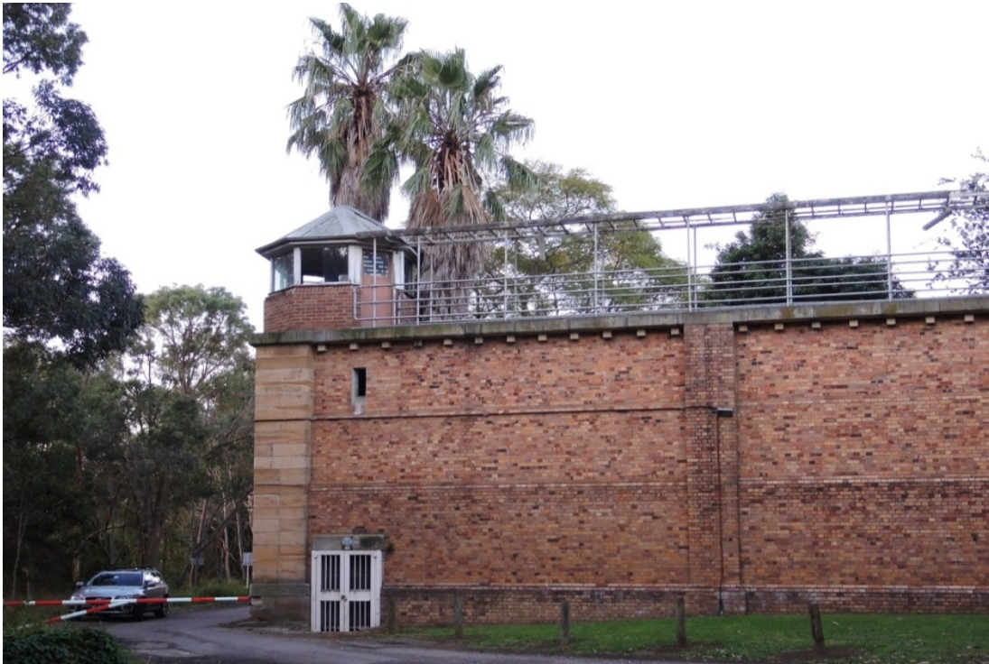
60 The high brick wall at the north-western corner of the Linen Service. Source: MUSEscape, October 2015.
