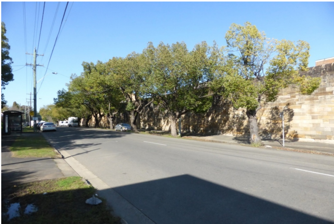
58 View south along O'Connell Street showing the Camphor Laurel street tree plantings outside the walls of Parramatta Gaol. Source: MUSEcape, October 2015.
