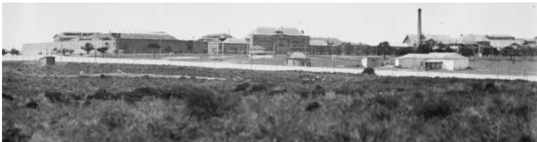
81 Panoramic view of Long Bay, 1932, showing its impact as a prominent landmark in the locality. Source: National Library nla.pic-vn6300247.
