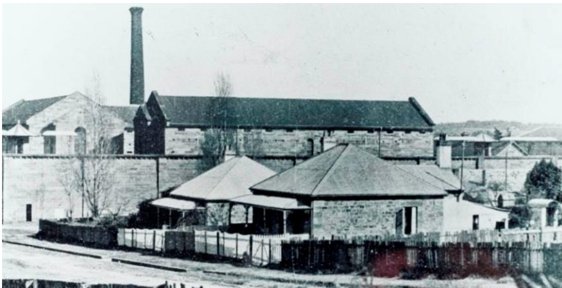
E-4 A c1911 view of Parramatta Gaol from near the intersection between Windsor Road (Church Street) and Dunlop Street. Development during the late nineteenth century has begun to impact views of the Gaol. This view is no longer possible due to the development along O'Connell Street, Dunlop Street and Church Street. Source: Parramatta Heritage Centre.
