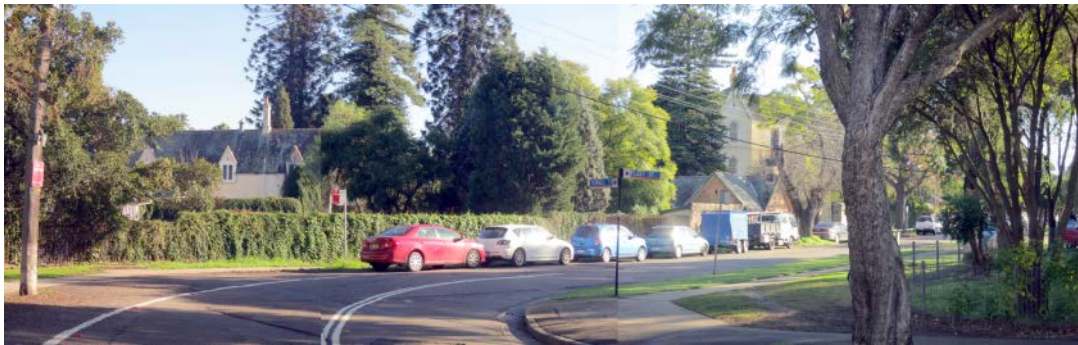
The view of the Norma Parker Centre/Kamballa buildings from Fennell Street (near the intersection with Fleet Street).
