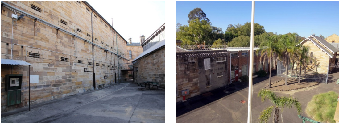
Views within one of the original triangular-shaped cell block yards, which generally feature high stone walls on two sides (left) and views within the original entry yard (right).
