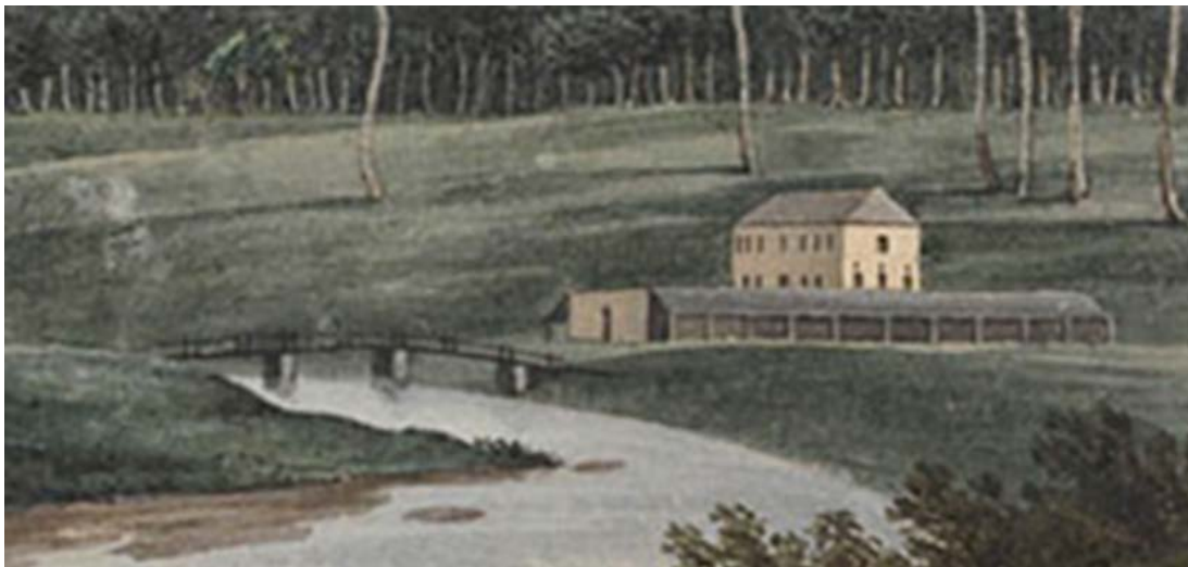
F-9 Detail from c1809 painting showing the gaol with second Factory storey and gabled roof, stone perimeter wall and gate, and two timber sheds with skillion roofs and possibly with open sides on the east and west sides of the wall. Source: ML, SLNSW (PXD 388).
