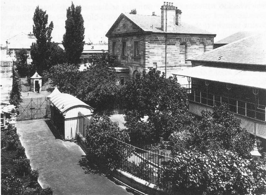
D-13 The forecourt of Parramatta Gaol c1889, at the height of arboreal excess under Governor Barnett. Security requirements resulted in a drastic reduction of vegetation in the new century. The palisade fencing was standard in NSW gaols at the time and gave an open feel to the area. Source: Department of Corrective Services.
