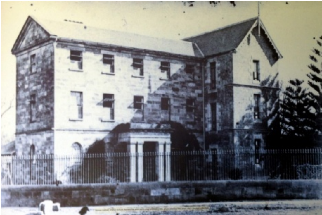
48 View of the main building c1870, after construction of the c1867 three-storey addition (north wing). Note the installation of doorways on the south face of the north wing—they suggest that a balcony was intended for the front (east) elevation of the building but was not implemented until construction of the south wing addition in 1882. Sources: Society of Australian Genealogists—Houison Collection.
