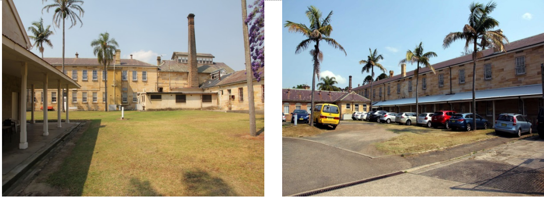
Left: The courtyard created by the former Third Class Dormitory Building (C105), Spinal Range (C107) and the Dormitory Building and Kitchen Annex (C104a). Right: the courtyard created by the former Spinal Range (C107), Ward 2 (C109) and the perimeter walls to the east and north.
