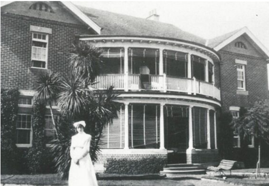
D-11 The former Nursing Administration Building c1920. Constructed in 1909 as an administration block and Sisters' Home, it served as Nursing Administration from 1970 until 1993. The front of the building faces the river but the historic visual link between the building and Glengarriff on the west side of the river has been lost due to construction of buildings in the 1990s. Source: SLNSW – bcp_01641.
