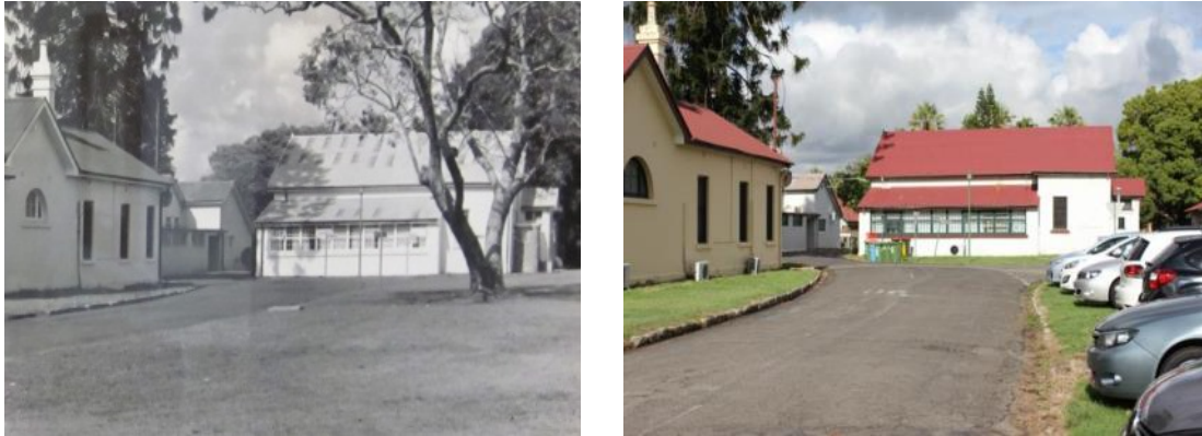
An earlier view of the former Female Asylum Kitchen from along Eastern Circuit (north) (left) and today (right).
