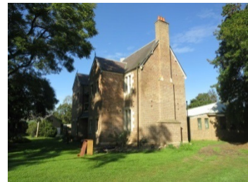
Bethel House on the Norma Parker Centre/Kamballa site
