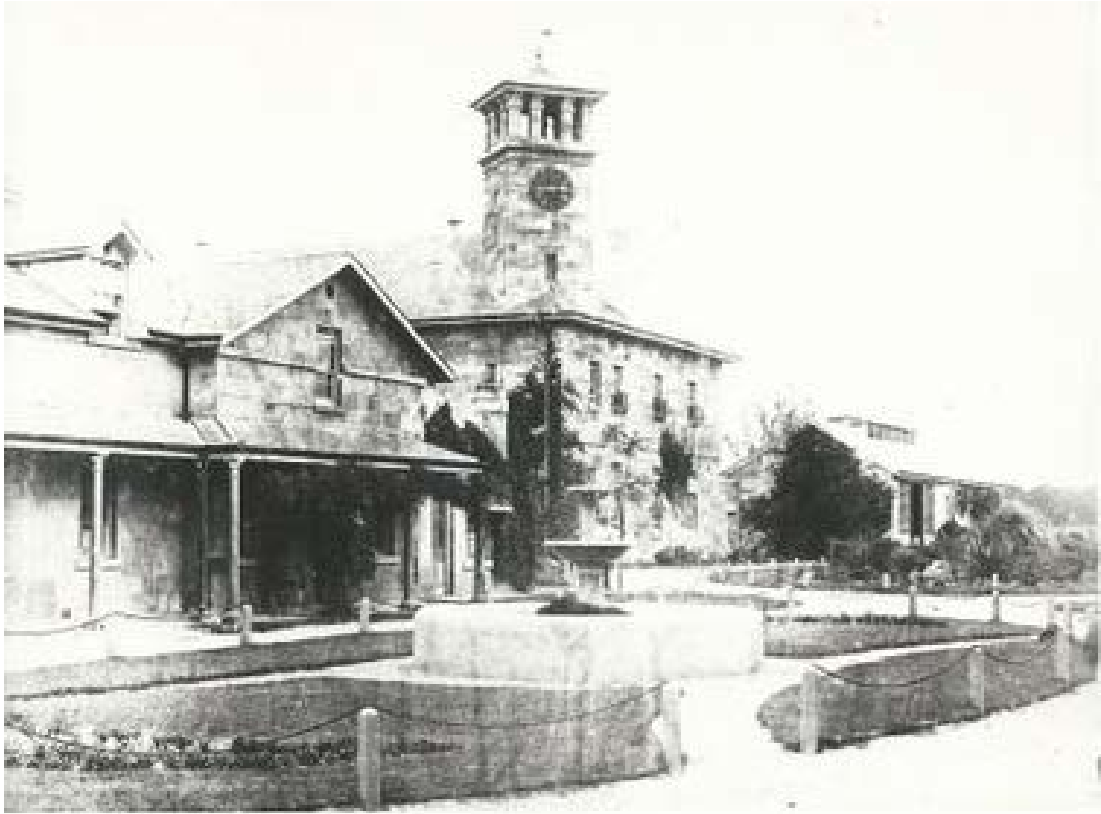
D-8 'Male Ward 1 and Main Courtyard c1888', with the 1884 building erected using stones from the Female Factory dormitory building and the dining hall behind. The southeast Range of the Female Factory is at the left.
