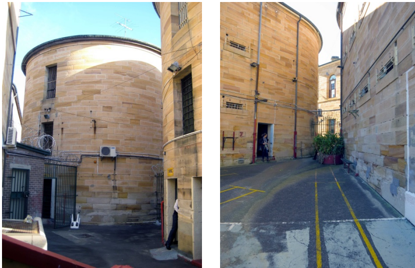
Views of the narrow spaces between the original three cell blocks and the Governor's House.
