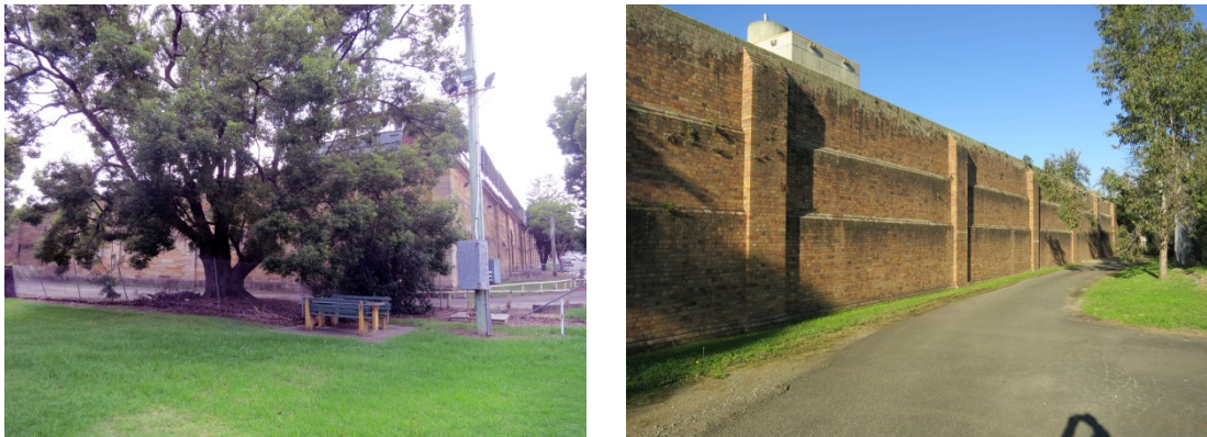
Views of the Parramatta Gaol walls from within the Cumberland Hospital (East Campus) site.
