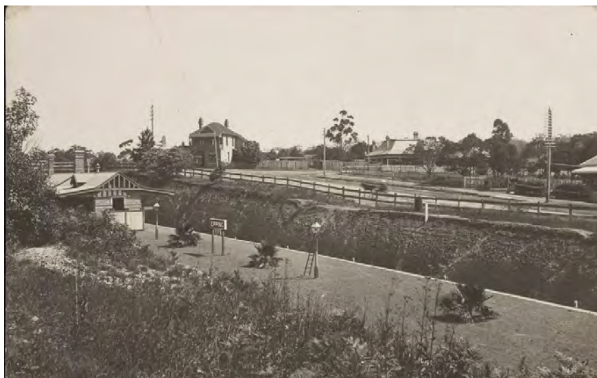
Figure 7: Epping Railway Station in 1906. The bridge which now forms part of Bridge Street is visible in the background to the left and current day Beecroft Road runs along the length of the image. (Source: National Museum Australia, Josef Lebovic Gallery collection no. 1)
