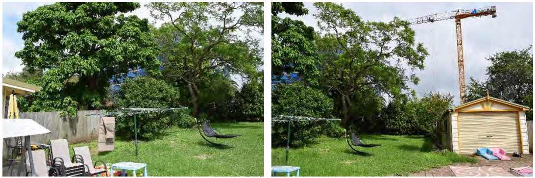
Figure 70: Views from the rear of 42 Essex Street, a heritage item of local significance, toward the development at 20-24 Epping Road. As with 40 Essex Street, the high density residential development which is under construction lies directly behind the rear fence of the property, with minimal setback from the property line.
