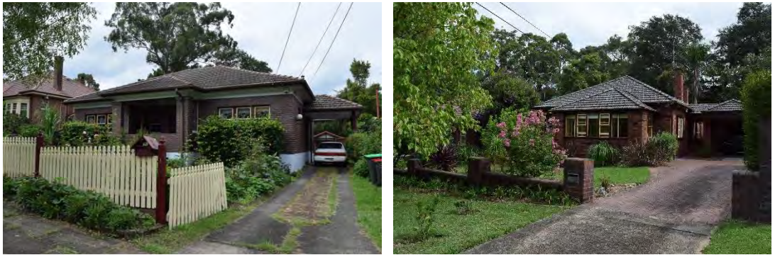
Figure 41: 16 and 17 Rosebank Avenue, respectively, are designed in an Inter War Bungalow style. The Bungalow style is featured the most amongst the dwellings of Rosebank Avenue
