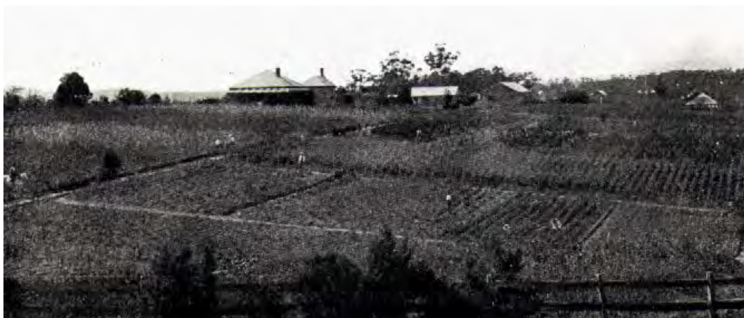
Figure 8: View of Mount Tomah nursery in 1902, possible looking from the crest of present day Pembroke Street, looking south. The two dwellings on the left-hand side of the picture may possibly be 42 and 46 Essex Street, both of which are dwellings which date to the Federation period, despite their current later additions. (Source: City of Ryde Library, 4969553)
