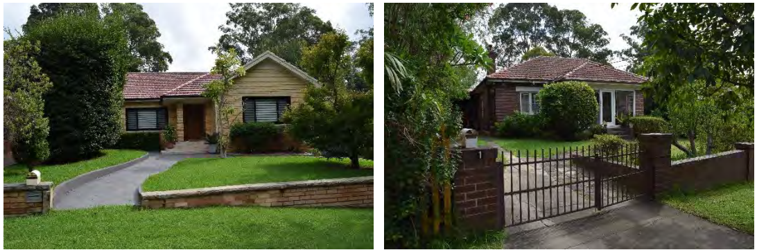
Figure 42: 5 and 1 Rosebank Avenue have undergone some modifications to the original fabric. 5 Rosebank Avenue has modified the entrance path and driveway, as well as the entrance way and windows, whilst 1 Rosebank Avenue has undergone some minor changes, including enclosing the front balcony and the installation of a new gate to the driveway. Despite these changes, both dwellings continue to contribute to the character of the area.
