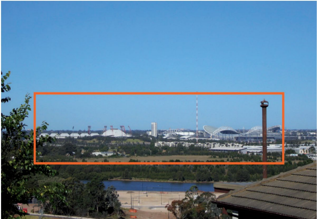
Figure A1.2.11 – Looking South towards the Homebush Olympic site, Coffey Street, Ermington
